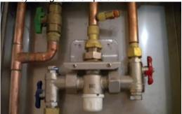
The *Legionella* risk associated with hot water systems incorporating TMVs may be reduced if the TMVs are in close proximity to the outlet(s) they serve, resulting in the presence of hot water ≥60 °C through the majority of the system.
